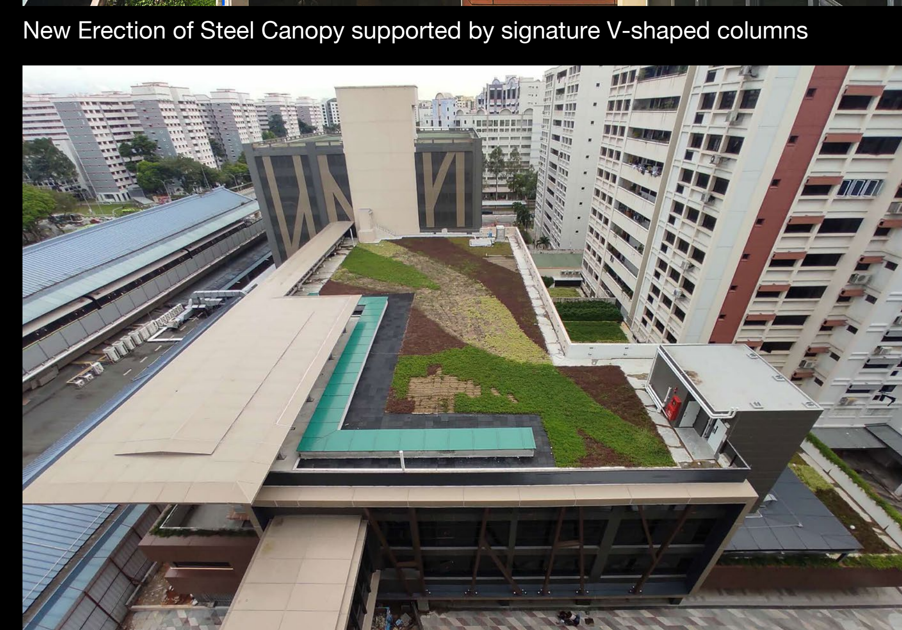
New erection of steel canopy and link bridge to Kampung Admiralty and addition of green roof
